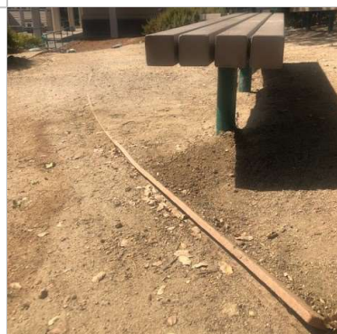
The edging along the path needs repair.
