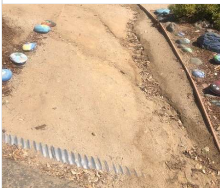
The decomposed granite on the path needs to be leveled.
